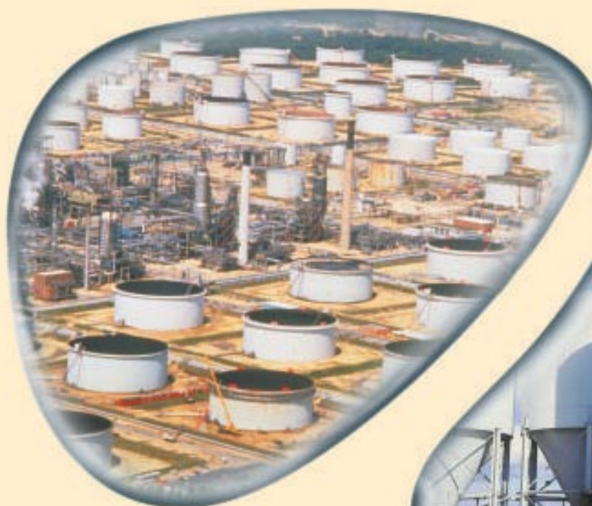
Inflammable gas storage.
